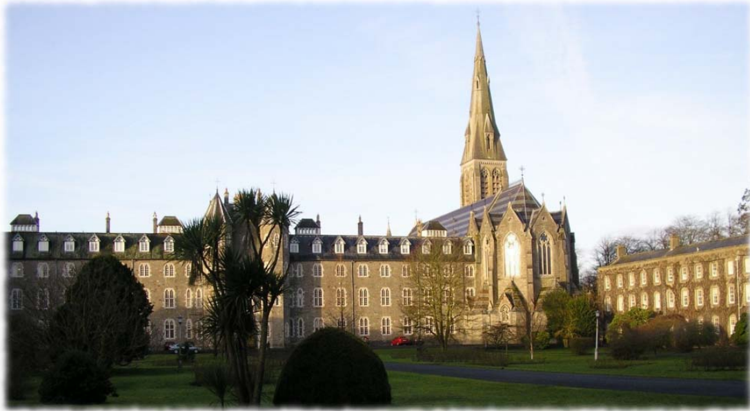
Saint Patrick's College, Maynooth, Location for the First International Workshop on Systems Biology, NUI Maynooth, July 2006
